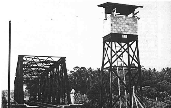
Below: A watchtower manned by Malayan Home Guards in order to protect a railway bridge. IWM
